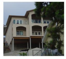
PILES EXTENDED TO SUPPORT DECK AND HOME BUILT ON SLOPES
