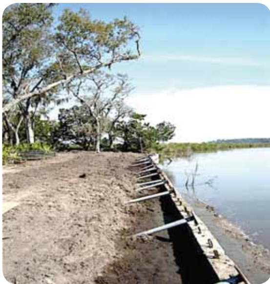
Figure E Retaining Wall Tie-Backs
