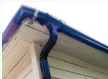
Poor repair of an eavestrough
