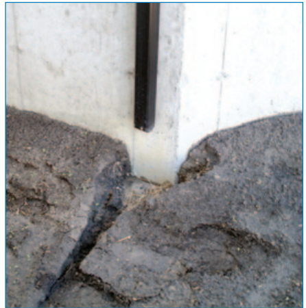
Downspout and grading problem.
