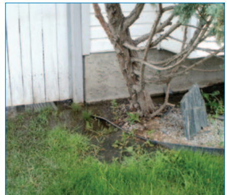
Water near a foundation.
