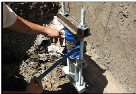
INSTALLING THE HYDRAULIC JACK
