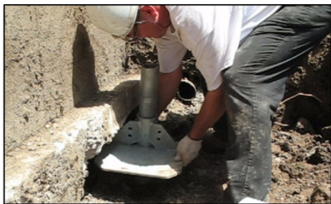
BRACKET INSTALLATION
